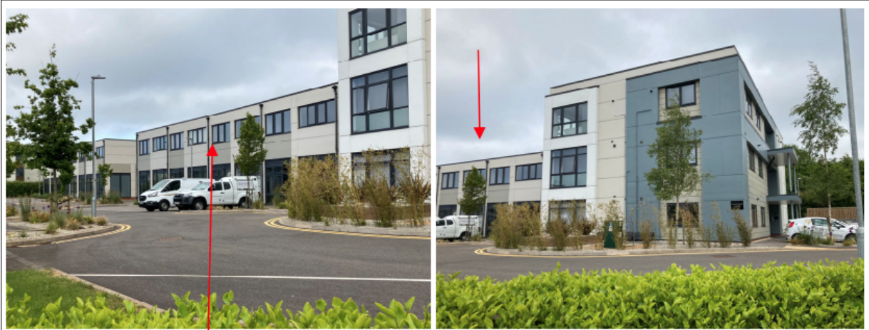
Block E looking from Hurricane Way in context with neighbouring blocks D & A
