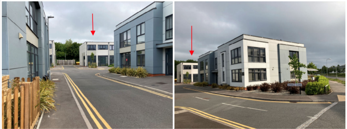
Block E looking along Spindle Close in context with residential blocks C and B
